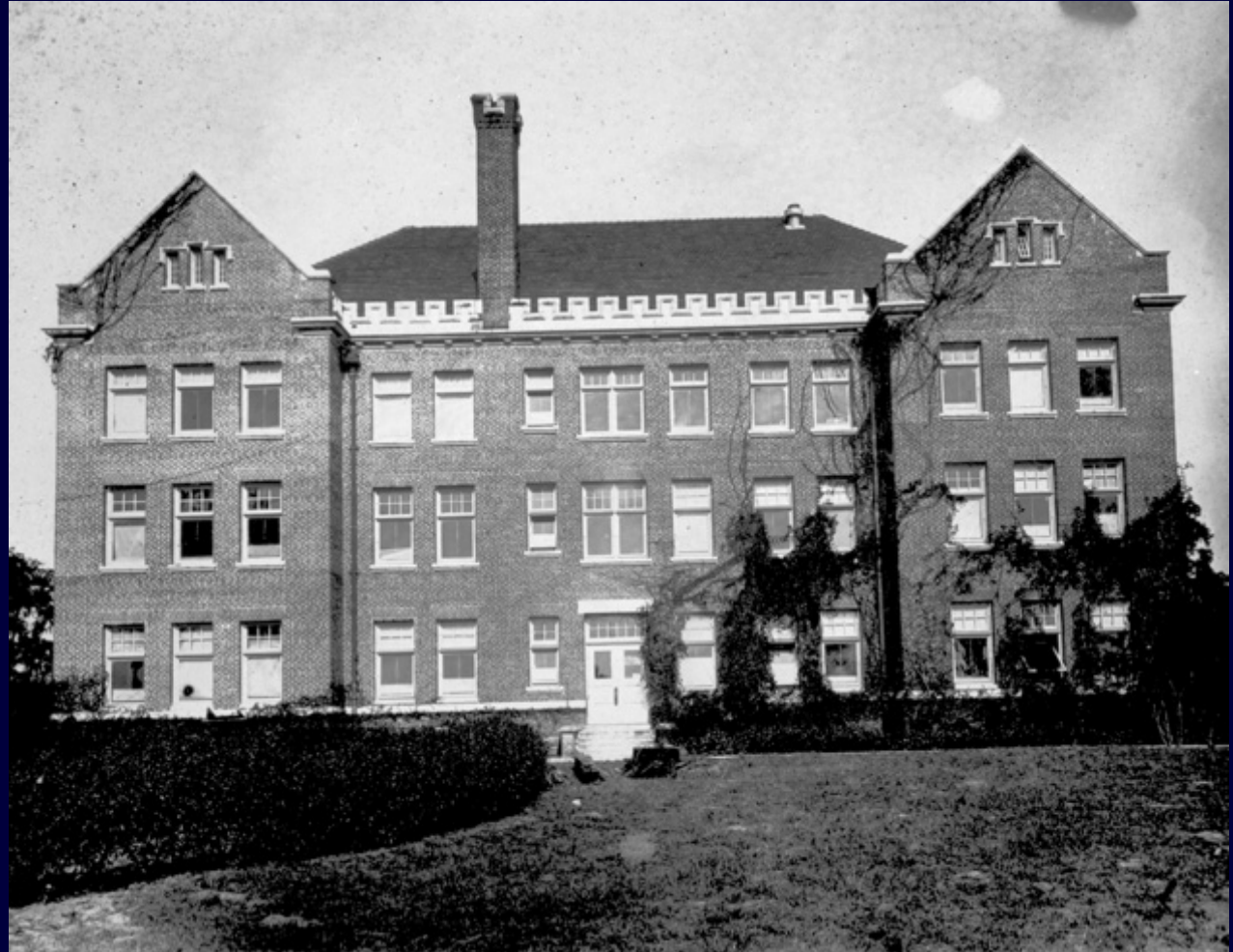
Early view (South Façade)
