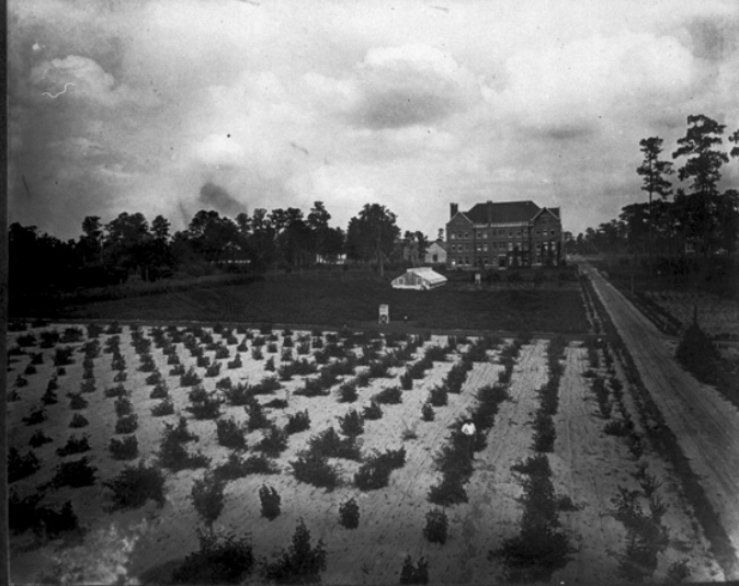
Experiment Station Hall. Plant Introductions in foreground.
