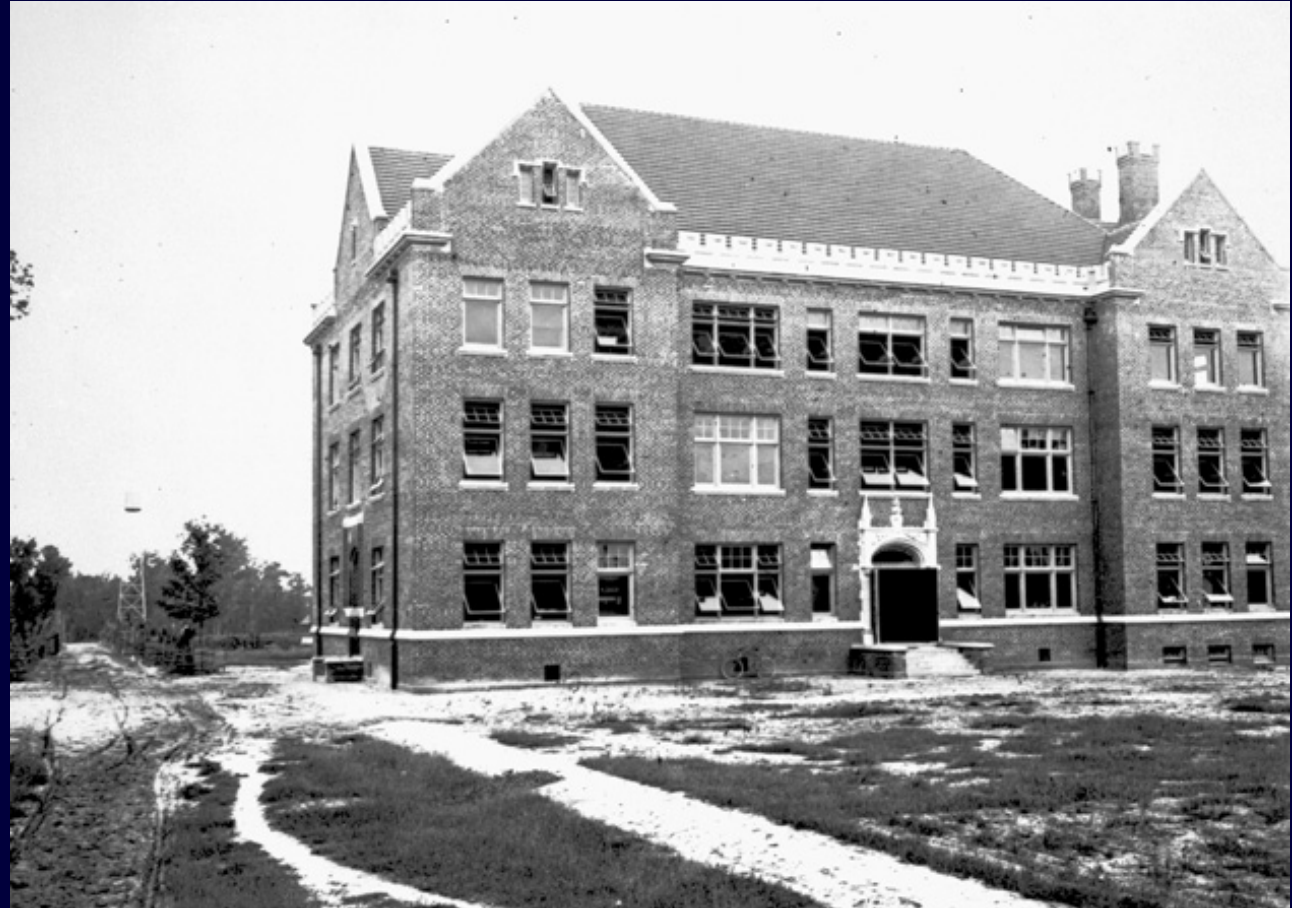
Early view of Newell Hall during construction
