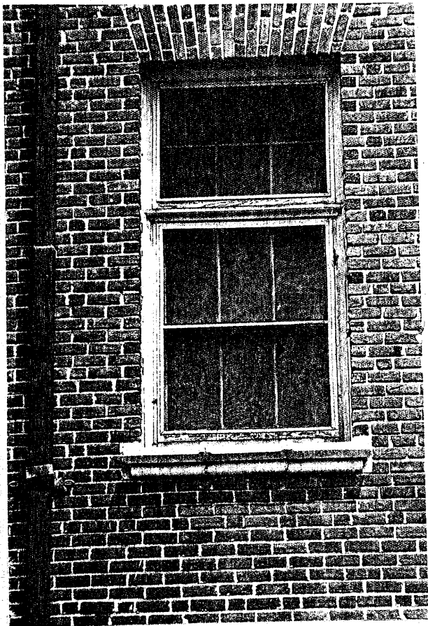
brick voussoirs and terra cotta sill typical window; south facade
